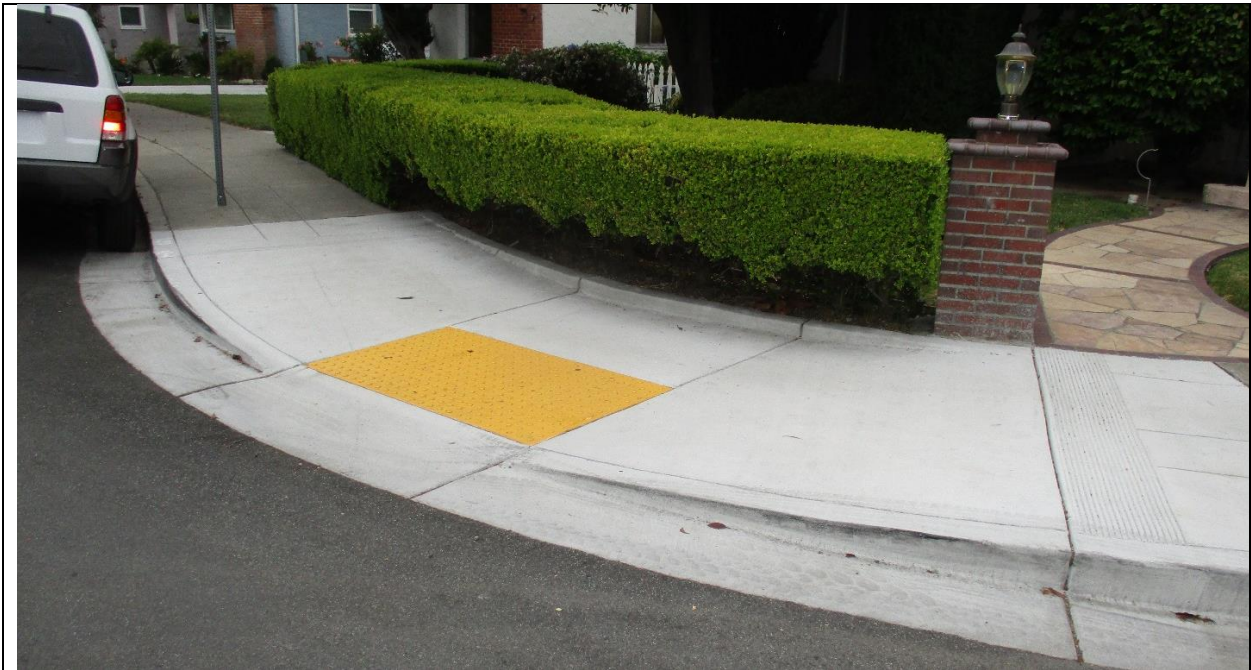
Curb Ramp Cherrywood Avenue
