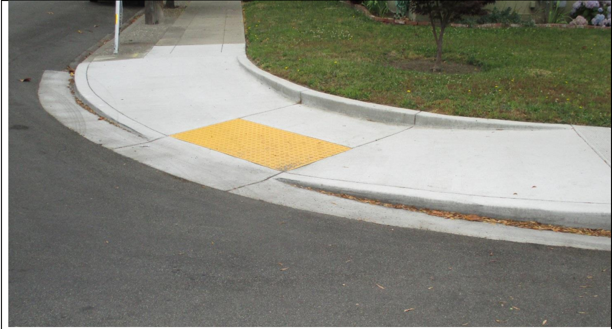
Curb Ramp, Leo Avenue
